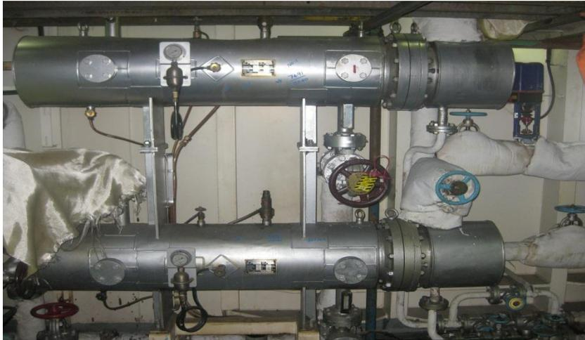
**Figure 7.4 – Typical fuel oil heaters**
